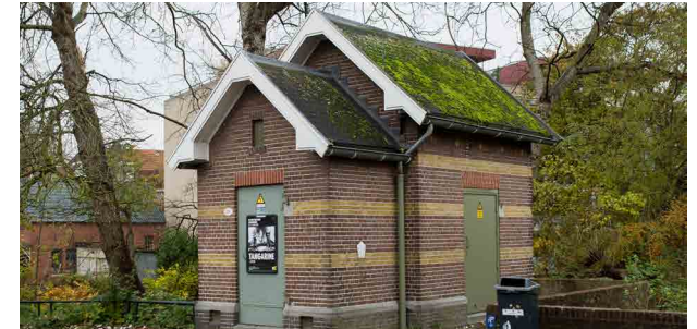
MS-MS station (3-23kV)
